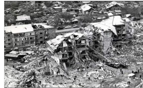
The Earthquake in Spitak in 1988 (Armenia)
